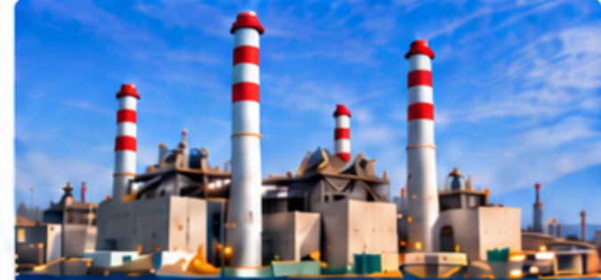
Jeddah South Thermal Power Plant
